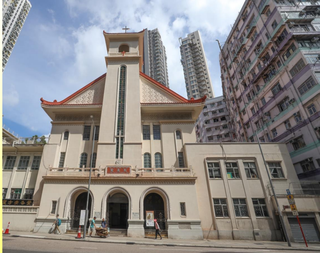
面向石硤尾街的正立面 Front elevation facing Shek Kip Mei Street
